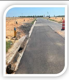
The damaged section of road from the fire hydrant has been repaired.
